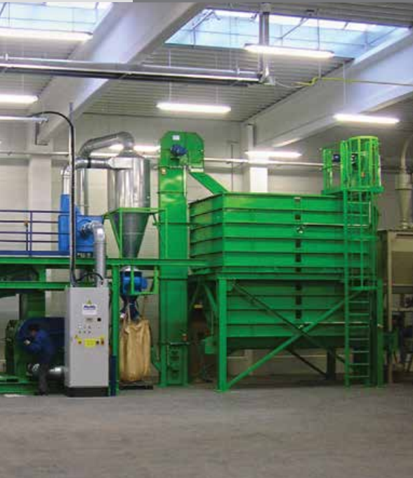
Hungary plastic waste processing plant
