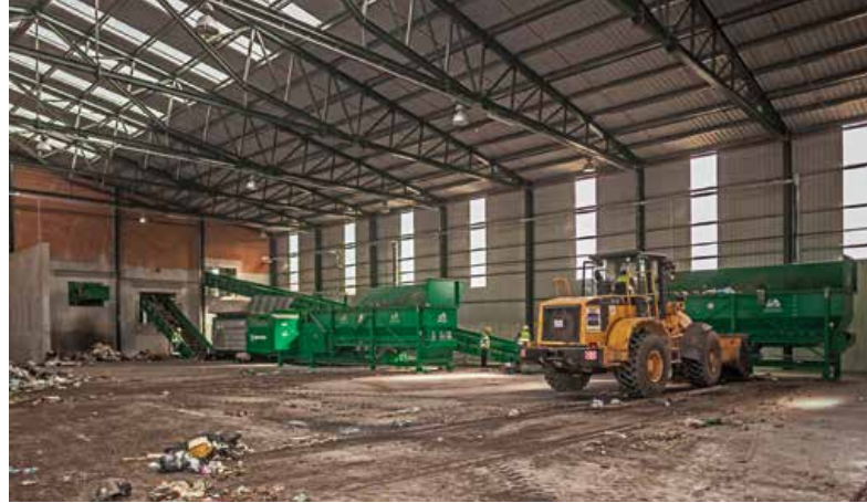
Waste reception building
